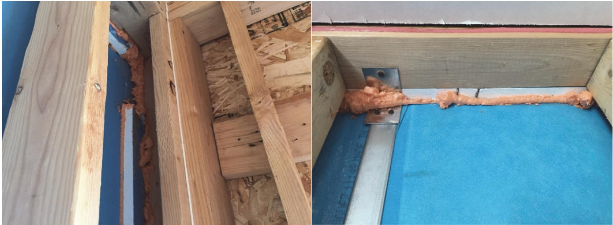
Figure 18 Air sealing for wood-frame construction.
