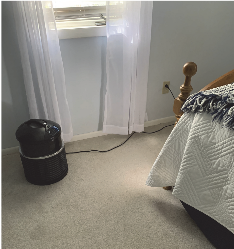
Figure 12 Typical use of a portable air cleaner device.
